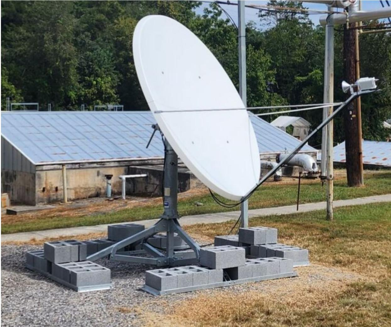
**Figure 5. Final orientation azimuth and elevation for the 2.4 m KU-band dish.**
